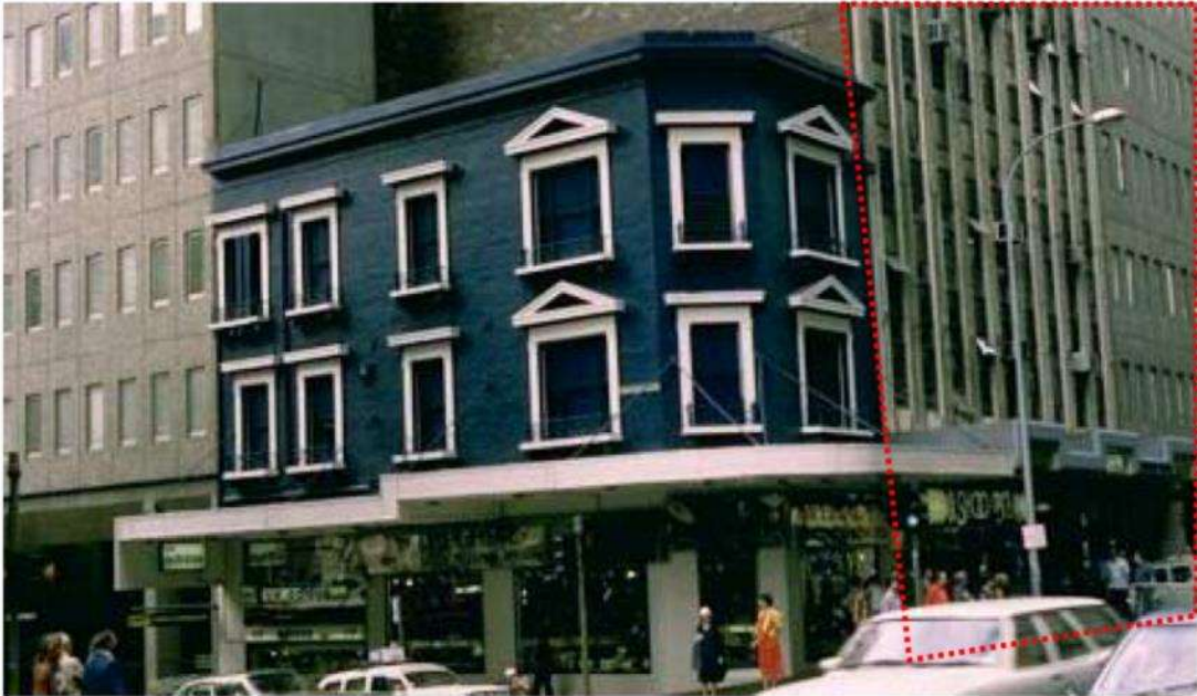
Figure 6-27 – A photograph taken during the 1980s showing remainder of building along George Street now demolished. Source: Department of the Environment and Energy rt08961 with GML additions.
